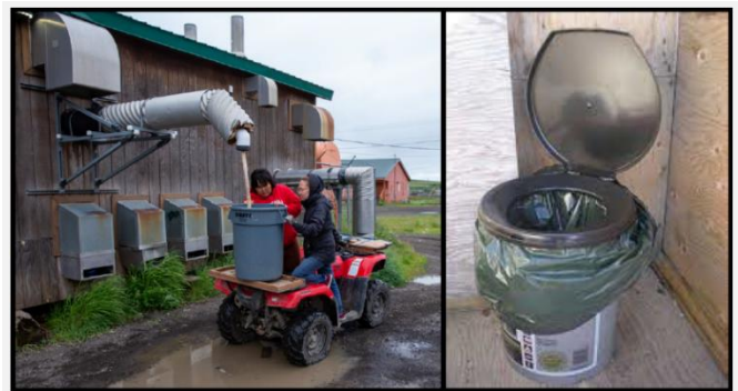
Figure 3. Village Infrastructure. Many residents of Stebbins, Alaska use washaterias (left) and honey buckets (right) for water and sanitation needs. This is common infrastructure in remote Alaskan communities.
